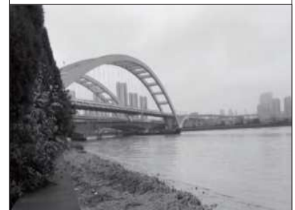
deformation monitoring of bridges and tunnels
