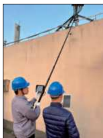
constructure inspection (WiFi real-time image transmission)
