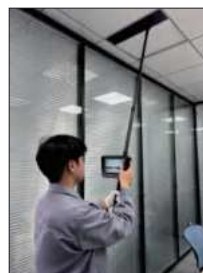
ceiling duct inspection
