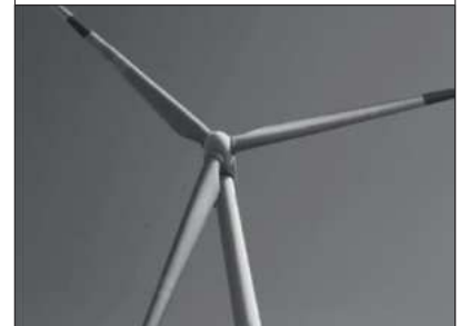
wind blade deformation inspection
